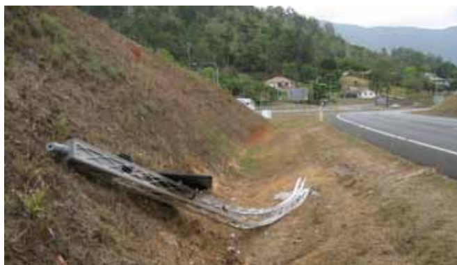
Figure 20: The driver of a vehicle travelling on Reservoir Rd, in a suburb of Cairns, lost control, spun and slid sideways into a Lattix sign post. No-one was injured in the accident. Photo courtesy of ASP Group Pty Ltd
