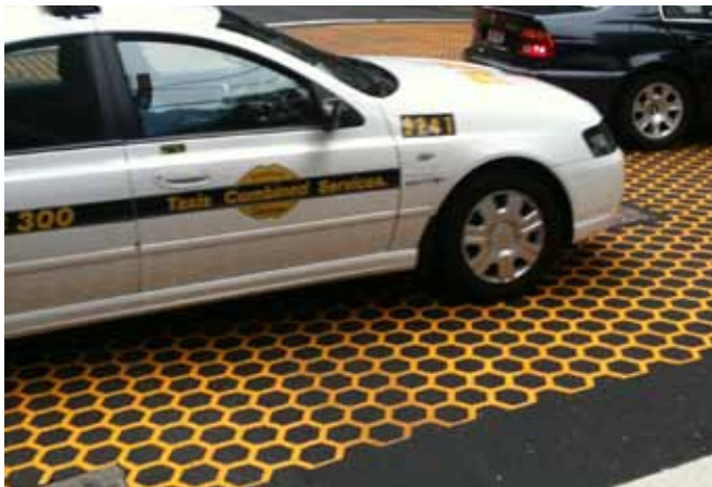
Figure 3: Example of queuing across new yellow markings at George/Hunter Streets, Sydney CBD. Source: NRMA Motoring & Services 2011
