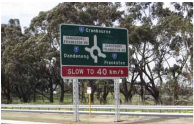
Figure 19: Example of Frangible sign recently installed in Victoria. Photo courtesy of ASP Group Pty Ltd
