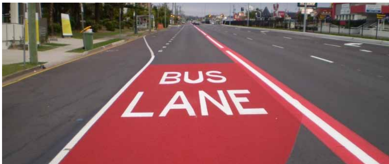
Figure 14: Example of painting only the start of the bus lane in red, and also painting the line separating the bus lane from the adjacent traffic lane. Brisbane City Council has adopted this approach. Source: Safe T Surfaces (STS) www.safetsurfaces.com.au
