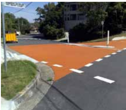
Figure 11: Orange Road Pavement Source: Safe T Surfaces (STS) www.safetsurfaces.com.au
