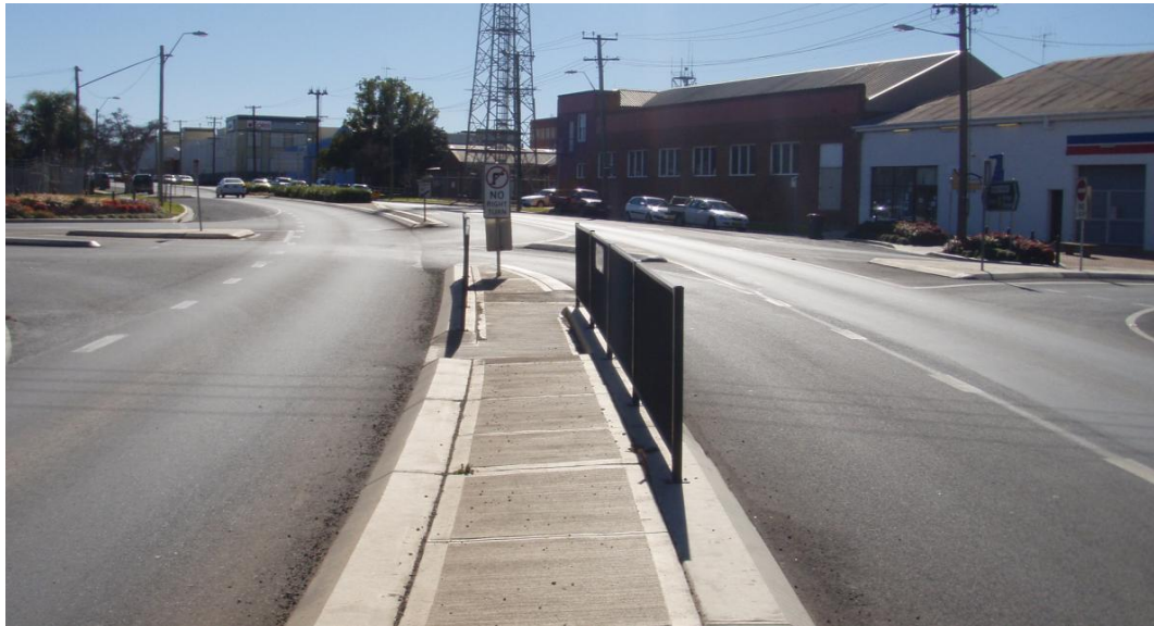
Figure 4-19 The Newell Highway at the Dalton Street intersection
