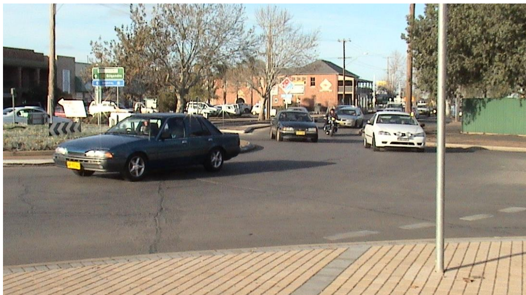
Figure 4-14 The eastern approach to the Newell Highway/Darling Street roundabout providing two-lane entry into a one-lane roundabout.
