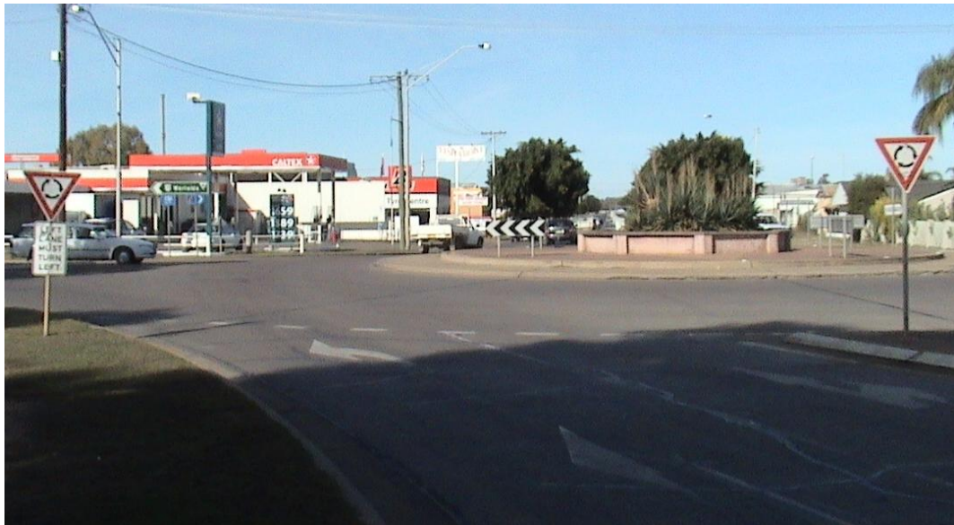
Figure 4-12 The northern approach to the roundabout providing two-lane entry into a one-lane roundabout.
