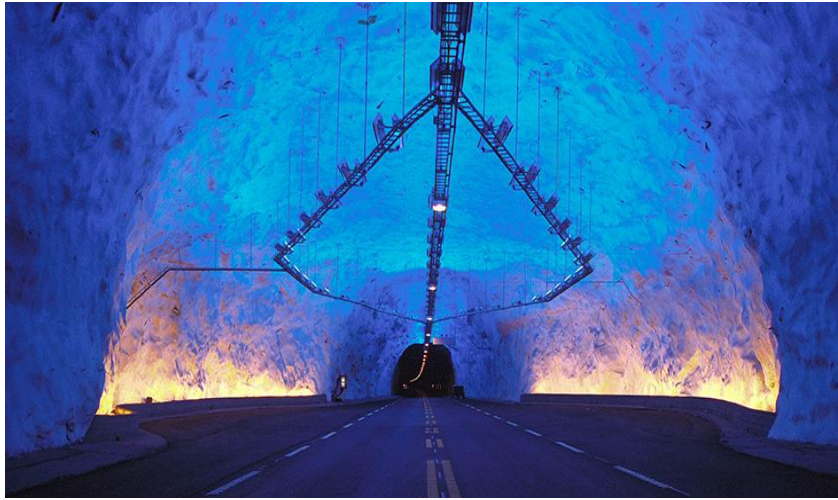
Image 1.7 – Image of the Lærdal Tunnel, Norway
