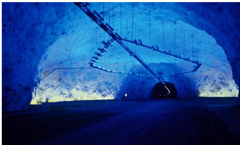
Image 1.6 – Image of the Lærdal Tunnel, Norway
