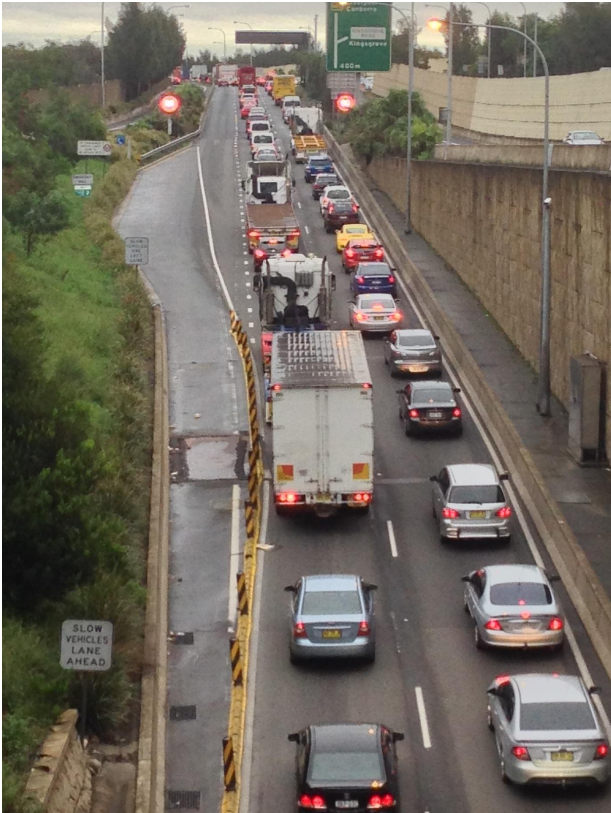
Example of existing traffic congestion on the southbound exit from the two lane M5East main tunnel at Bexley North in the PM peak.
