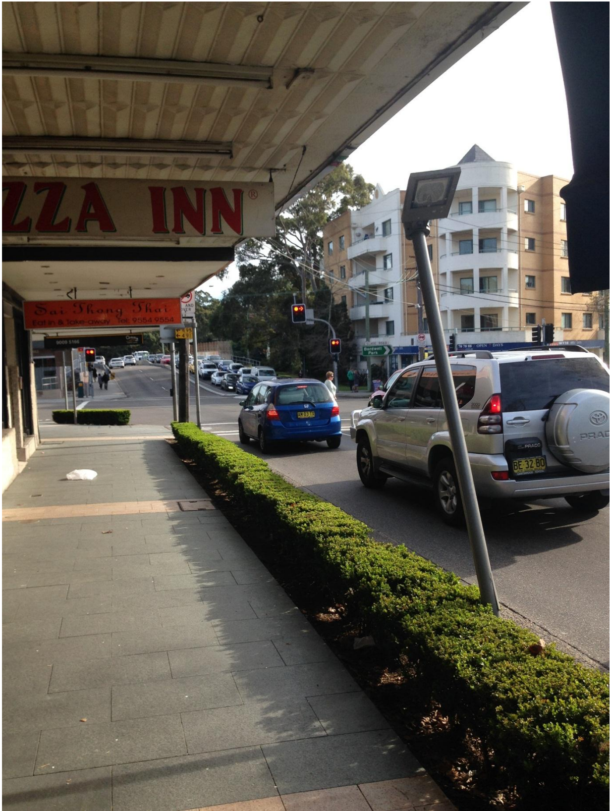
Example showing pedestrian light pole that has been hit on the Bexley Road footpath approaching Shaw Street and the proposed WestConnex construction site at Bexley North. The low hedge provides no protection for pedestrians using the footpath and errant vehicles changing lanes at this location have previously crashed into the adjacent pizza shop.
